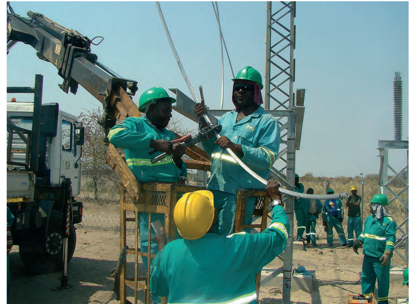
Construction team doing finishing touches at the Omuthiya 132/22kV Substation.
