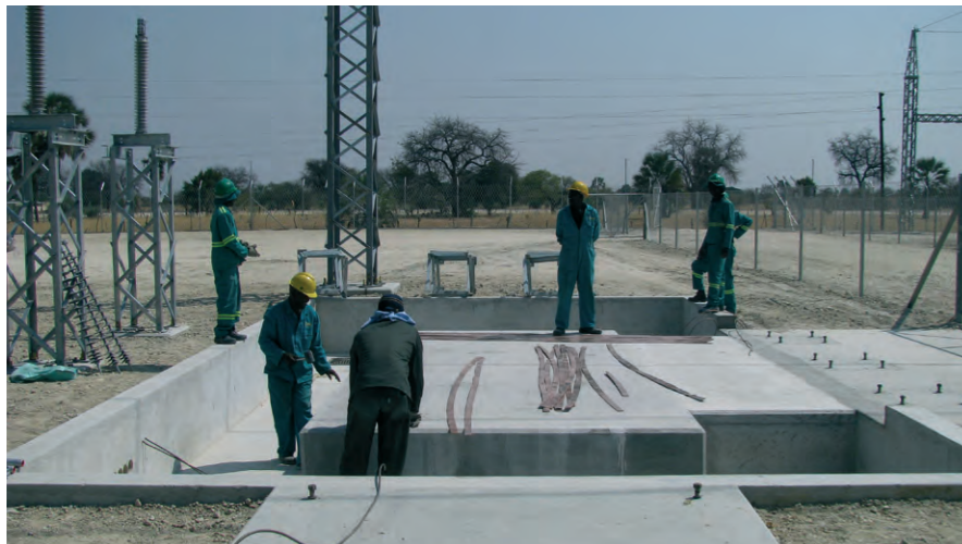
NamPower staff working hard to complete the Efundja-132kV/66kV Substation near the town of Helao Nafidi in the Ohangwena Region.
