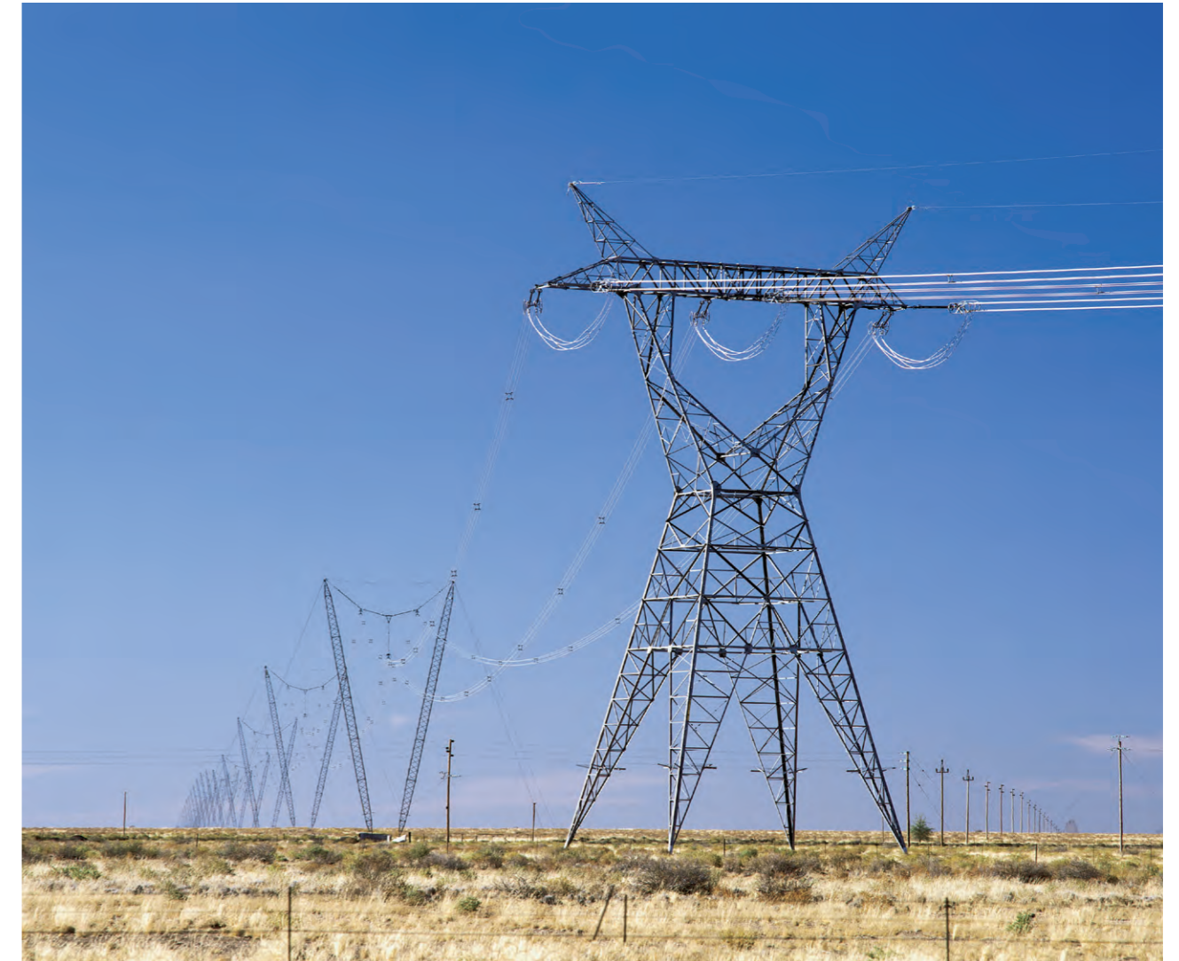
The 400kV line in southern Namibia is among the few transmission lines that are already fitted with OPGW.
